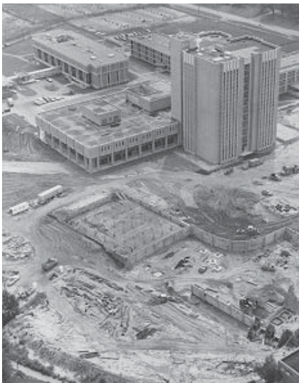
Student Center Construction, 1971
