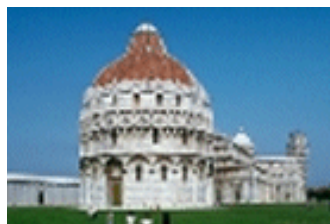
Overall view of complex from behind Baptistry
